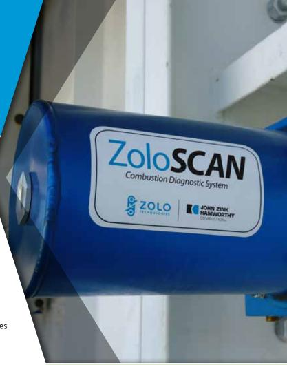
ZoloSCAN SensAlign heads (above) automatically realign. ZoloSCAN's interface (below) shows average data for each path and constituent.
